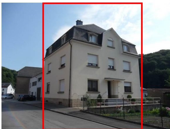
8, rue du Village – volume principal
